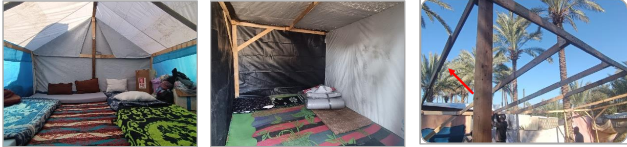
Figure 3 Using folded tarp pieces under nails HEKS/EPER July 2024
