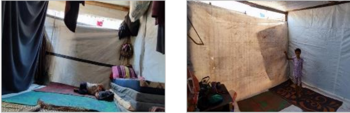
Figure 6 Leaving an upper air gap to improve thermal comfort (Source: HEKS July 2024)
